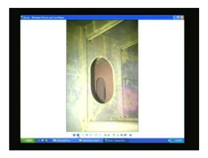
This is actually a picture of you can see from one this thing opening you can see some other member inside. It is like this, it is a case of what you call a floor, bottom shell longitudinals, struts and here this perpendicular to the plane of this if you can make out this inside red one; that is a side girder.
