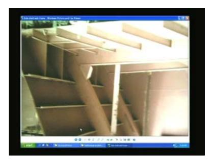
That means it should have enough life. So, they will protect the steel from the further corrosion, rusting till construction is over and give it a final coat of paint. Well these are some of the closer views. Here is the side shell longitudinals, it is a longitudinal framing system this is the side shell is of ford part which is becoming v. You imagine the forward sections of the ship.
