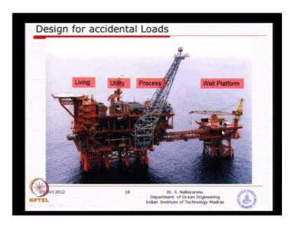
You see here this particular project where, the well plat form is on the right side kept separately because, this is a gas field and the potentially most of the time or 99 percent of the time, gas well platform will not be combined with the process plat form. If it is the oil platform, there may be potential chances of combining this with this, but never if it is a gas plat form, because of high potential of fire.
