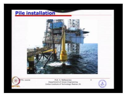
So you will have connection between this to the barge which is supporting the hammer itself which is what you will see if you go back to this you can see here several numbers of hoses going down to the barge, barge is actually at the background. So which will actually send the pressurized fluid which will make the annual hammer to lift it up and drop it, hammer is nothing but a heavyweight steel which needs to push up and down we have several types of hammers which we will see later part.
