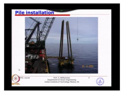
You can see this particular picture is a 4 legged jacket, what you see is 4 piles are just put on top of this jacket the reason is very simple. For example if I want to drive 4 piles, I take first pile 1 and drive, remove the hammer because every activity is involving crane, crane is the one that is taking the pile or taking the hammer. So every time when you want to change the hammer on pile it takes 3 to 6 hours.
