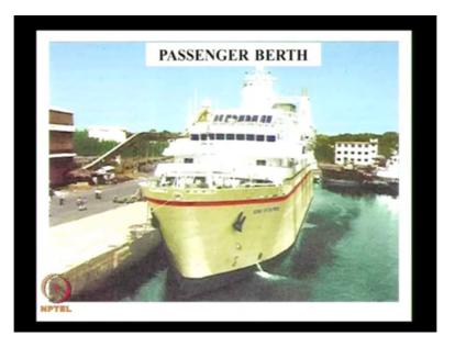
Here you have the access to the city very close by and this portion is the pith of the structure which is designed for heavy loads is the backup area. So we will be discussing about design of this portion which is called as the Apron.
