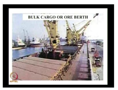
This another example is bulk cargo or over berth which I have taken here this is the ship and you have the hatch cover the crane is in the ship itself called as the self geared vessel. So you take the cargo from the ship and then put it on a chute here through which it can go to a tipper and it can directly move. So this is a bucket which is used to grab the cargo and put it here. This is the berth the crane is not on the berth, the crane is on the ship itself .
