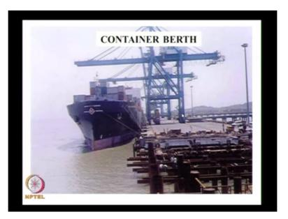
This is a typical container berth this photograph is taken from Jawaharlal Nehru port this is berthing face there are approaches here there is a high mass tower here. The vessels will be having containers may be three stacks or 4 stacks or 6 stacks in the vertical direction. This is a ohm so we can lift the container take it here and drop it to the waiting truck. The waiting truck will move away what you are seeing here is a construction which is going on for the extension.
