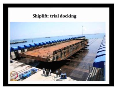
Shiplift for trial docking, this is the photograph from L&T Kattupalli project. They have commissioned in 18 months time. These are the haunches. This is the end-haul pattern.
