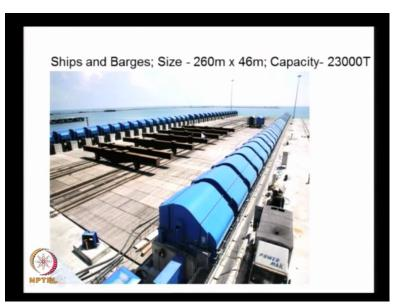
This can handle ships of size 260 meter by 46 meter. The light ship weight will be about 23,000 tons.
