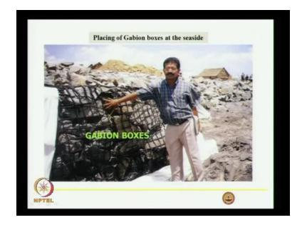
I was telling about 3 metre. This is the 3 metre width. And then they will put another 3 metre here, they will overlap here 300 millimetre. This is the sea side. Whatever sand they are excavating here, they have it as a core stone dam here. They have put the gabion boxes. Originally we have taken the filter fabric on top of the gabion box. Finally we found that it is not good. It is not as good in ultraviolet protection as before and does not allow the dissipation of waves also.
