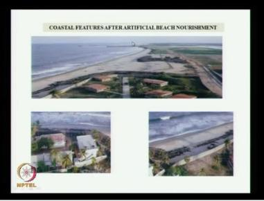
So here you are seeing this photograph again. This is your south breakwater and this is your north breakwater and between them, you have a submarine tunnel. You dredge it here and then through the submarine tunnel, it comes. See, able to see the pipeline here. Through the pipeline, it comes and it deposits. What you are seeing here as rubble mound seawall, it is also seen here, rubble mound seawall, these are all the places up to which the shoreline was there.
