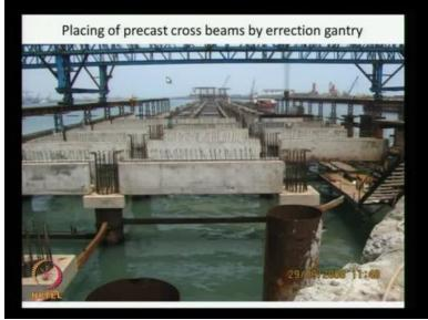
And this type of gantries which is made of 30 metres running on the rails is also essential. So once they complete this piles, pile caps and precasts units like this, then they can pour the
