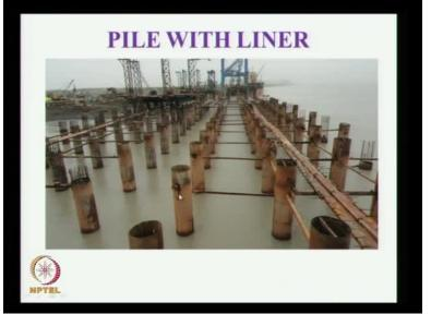
Now we are seeing the liners which have been completed. Earlier days, they used the liner also by gantry. Gantry means there is a platform for which we have the piling rigs. This is used to drive the liner. In this particular project, they have a floating barge using which they have completed the liner to make it faster. These are the bracings that has been made to connect at the top providing stability. Once they complete the liner, they provide the reinforcement inside.
