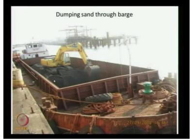
This is the barge which is used to dump the sand which is taken from elsewhere, from an airway berth they will take it on a barge and take it very close to the berth under construction and fill it.
