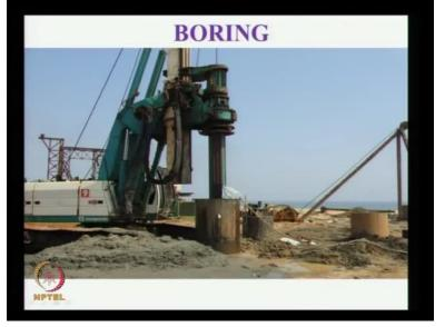
You are seeing one tripod here. This is a conventional wench is used, this is time consuming. Whereas this is called as a rotary rig which will drill through the liner. Typically, the liner is about 6 millimetres in thickness. It is rolled from a plate and made a circular section and we make in 6 metre or 3 metre pieces and then build it circumferentially. Each liner plate is welded longitudinally also.
