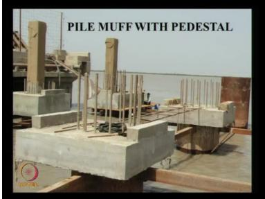
So here, you are seeing this precast pile more. There is a opening here inside which will be done in situ concreting. There are some pedestals which are projecting above, this is used to support the cranes. You are seeing another pedestal here. This is to support the beams. There are 2 beams, one is the crossbeam, another is the longitudinal beam. Crossbeam depth may be more and longitudinal beam depth may be less.
