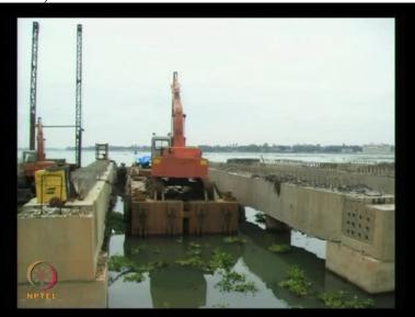
In this figure what you are seeing is a dredger which is dredging in between the main crossbeams. There are piles below this. This side is the landside and that side is the sea side. I will tell you why we have to go in for this type of dredging.
