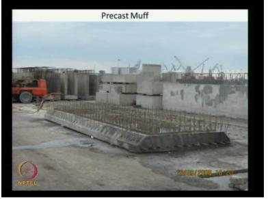
Here we are seeing the deck element. There is a (())(21:39) given here. So when you have the precast and in situ construction, there should be some integrity between the precast and in situ that is given by the sheer stirrups what is provided here like this. And this is how they stack it because space is limited and this is a U type construction which is made for the beams with reinforcement in between. So this cost is going under precast and inside what is going is in situ.
