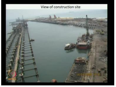
This shows a construction site at Chennai port. This is a 2nd container terminal. So we have typically about 4 rows of piles here, 1, 2, 3, 4, sorry 5 rows of piles. 1, 2, 3, 4 and 5. There is a tube which is transporting the, there is a walkway in which there are concrete is transported through the tube and we are see what we are seeing is the piles here, then we have the pile cap. And major time taken is for the piles.
