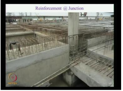
Here we can have the junction detail how the junctions are there from precast elements with the pile cap.
