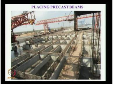
Here we get, this gives a better view where we have the place where concrete is being taken for in situ portion. This is a U type precast elements which are placed.
