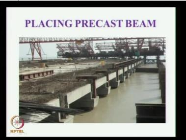
And here we are seeing the beams which are placed here and then the slab reinforcement, some concreting completed.
