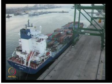
This is the finished completed we the 2nd container terminal. What you are seeing is a 30 metre span in which you have the rails which are fixed. These are the fixtures that is coming into picture. There are some Bullards which are used to tie the vessel and you may see some fenders also below the water level. This comes under wharf accessories.
