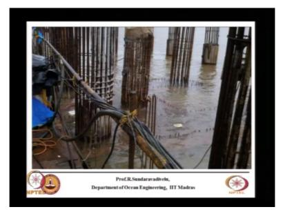
Bundled means two bars together they will keep it.Suppose you want to provide a 60 bars (()) (12:05) pile the spacing is 60. If you calculate the spacing it will not be less than, it will not be more than 100 millimetre clear gap, then you put two bars together bundle that means you put only 30 bundled bars. Each bundle containing 2 bars you can have 20 bundles of 3 bars in each bundle that also you can do.
