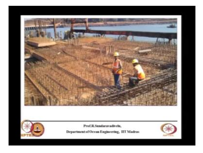
So once you place the beams precast then you put some top reinforcements when they put these precast slabs so we will discuss in the next class about the design of slab.
