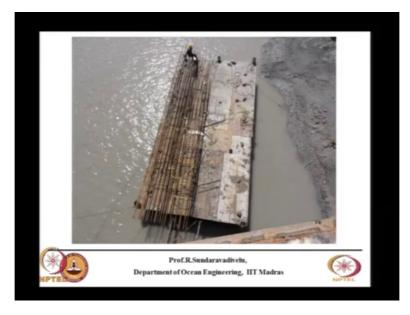
So this is a reinforcement bar which is transported by a barch. What is the length of (ba) reinforcement that is available in the market? 12 meters hmm? 12 meters, so if you are handling a 12 metre long bar it has some weight it may vary from 3 tons to 6 tons depending on the reinforcement. You are seeing some inner rings here may be in another fear it will biz in. This is to keep the bar in position.
