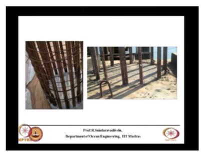
So here what is shown is I do not know whether you are able to see this clearly this is the inner core of the pile and this is the main bars this may be a lap bar or it is a bundled bar what you are seeing is a pile cap which is coming and sitting on the cover of the pile reinforcement. What you are seeing here is a pedestal and these are the hooks which are provided to lift the pile cap. So this is type of construction which they do generally to speed up the construction.
