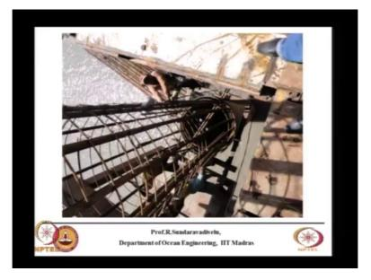
There is a person who is holding the bar and is lowering it for, lowering these bars also we need to provide some hooks and other things, it is not shown in this that also is a part of the temporary design. Here you can see the larger diameter this is your inner bar and these are smaller diameter bars which are outside. These are the main reinforcement bars.
