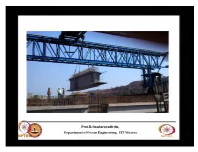
So this shows how they are doing the installation this is how they are lifting you have the hooks here then you are lifting it. So there are two stages of design one is for lifting what is the reinforcement required actually it is not done like that what they do is they do for the final stage of loading find out what are the reinforcement provided at the bottom and check whether that reinforcements are sufficient during lifting.
