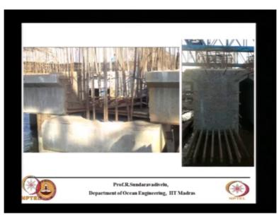
This shows another view how they are placing these bars specially the bars you can see here. This is for the sagging moment same calculate you calculate or use this formula to calculate the percentage of steel then provide the percentage. You have to provide some minimum percentage. What is a minimum percentage required for column? Column is 0.4 percent pile is 0.8 beam is 0.2 percent this is minimum reinforcement which you have to provide for the main bars.
