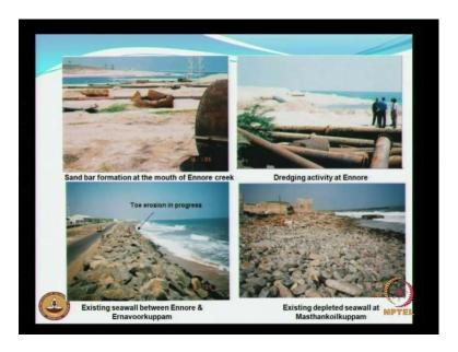
So, some of the other problems; see closure or river mouth, sand bar formation etcetera, around the same stretch of area. So, how the sea wall has failed? Because of, look at this, the toe erosion starts. Once the toe erosion starts, then that is a problem. Then, toe erosion continues and the stability of the stones become questionable and the whole thing collapses.
