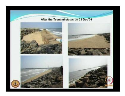
After the tsunami, you can just see, the 28<sup>th</sup> December, some of the locations were still there with the sand. Tsunami did not remove the entire sand. In some locations, the sand was there and the groins really sustained the tsunami because, there is not much of problem with the groins. So, I will come back to the effect of tsunami when I talk about tsunami interaction.
