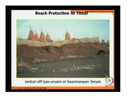
The beach protection that is to be done is for this kind of a scenario. So, you can see the kind of erosion that has taken place, the erosion is almost like vertical cuts and this needs to be protected.
