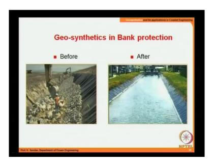
So, this is adopted for the bank protection. So, bank protection is going on. So, you see the geo textiles already laid on the sides. The side has to be prepared, there should not be
