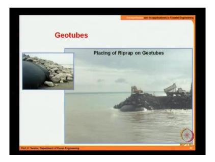
So, this is, this figure shows how the geo tube is placed and then in order to protect the geo tubes then you have a, you have the stones, dumping of stones is in progress in both the, in the, in this picture.
