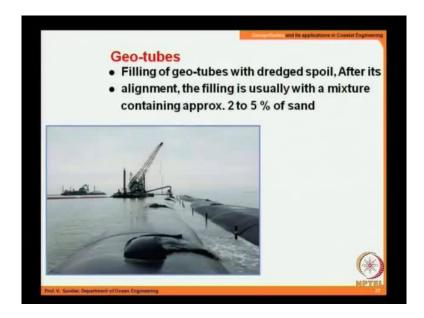
So, filling of geo tubes with dredge spoil. After its alignment the filling is usually with a mixture containing approximately 2 to 5 percent of sand. So, the water will come out as I said earlier. I also mentioned that we call it as a tube it is circular, but after filling you look at the shape it takes. So, it takes something like the shape of an ellipse and you can now this looks like a solid obstruction for any and it can resist forces due to waves or currents.
