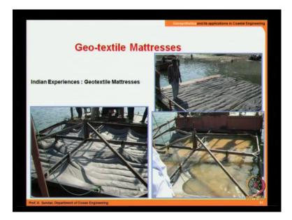
About close to the same location you have the installation of geo-mattresses. This is particularly helpful or useful in the case of leveling and also making sure, that the soil is being retained from erosion.
