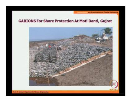
Gabions are, as I told you, is also very, very nice way of protecting the coast and you see, that here you have geotextiles, geobags, that geobags act as something like a cushion and geotextile prevent the soil erosion, and this gives the resistance of waves and over which your gabions can be placed.
