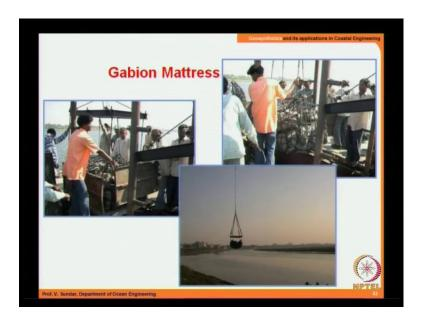
So, again this is the, how the geo-mattress is being laid there in the bottom on and there on the top you have lifting of gabion.
