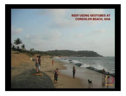
And then this is in Goa where you see the series of geo-tubes provided there. And if the same kind of the geotube is oriented just below the water level, it can facilitate a breaking also. So, this is a kind of another kind of concept that is being thought of or adopted.
