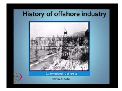
Similar thing happened in Summerland in California. You can see many of the drilling bricks can be installed very close to the coast to be at a shallow water depths, men essentially for oil exploration. Not one, you can see many of them as a cluster being constructed and elected very close to the coast in Summerland in California.
