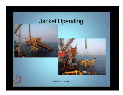
This is the process what we call as upending that is erecting the leg from on towing position to the upright position.
