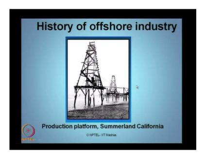
We can also see a photograph of a production platform which was simple as that which as trust system not one many of them resting on few of the legs may be six legs in this case as well it is got a depth they got a trust they got a supporting system located in a shallow depth because the structural system appears to me as very simple. So, is one of the production form which is be in photograph in Summerland California.
