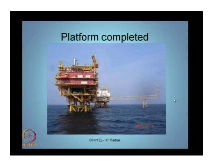
The plat form is now complete is what we have one of the classical jacket structures, which is fixed offshore structure in Bombay High Court.
