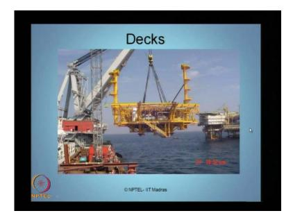
Now, the deck is being transported which is pre fabricated transported to get placed in position for the platforms.
