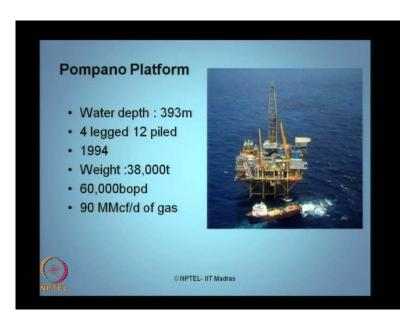
Let us look at the next platform. The photograph shows here a pompano platform; constructed at the water depth of 393 meters. It rest on four legged, 12 piled structural system; constructed in the year 1994. The total weight of the structure is about 38,000 tons, and this produced about 60,000 BOPD, which is equivalent to 90 MMcf per d of gas
