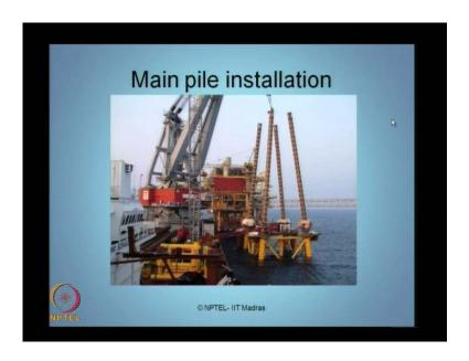
Main piles are getting installed for supporting the deck.
