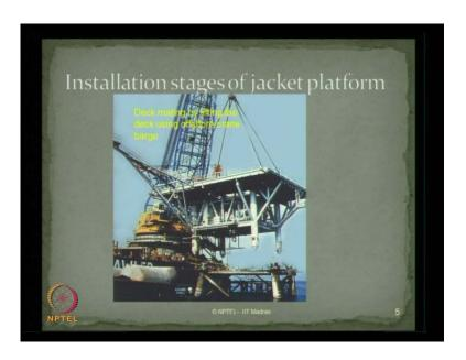
Once the pile is driven and the bottom is stable then the top side is being installed what we call deck mating. The deck mating is done by lifting the deck using an offshore special type of green barges, which is installed on the bottom structure as you see here.
