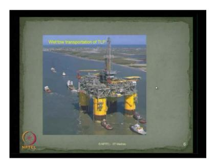
We can also do a wet tow operation of transportation. Now the figure what is see here show wet tow transportation of a tension less platform. So, this is the tension leg platform with top side details are see you here. So, these are all being guided by the duck board of lead barges and it is being wet tow to the site of installation.
