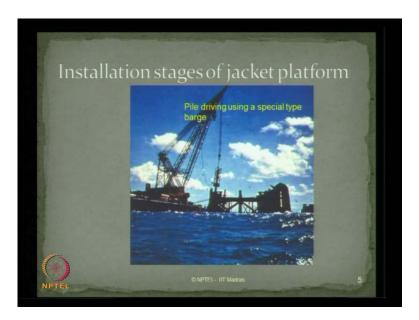
One side is tilted then the piles are being driven using a special type of the barge, which has got the loading capacity of the pile driving capacity here.
