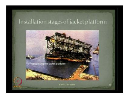
Let us quickly see, these different stages of jacket platform in detail. So, now, this photograph shows you the transportation of jacket platforms on a big barge as you see here. This is the jacket structure which being transported.
