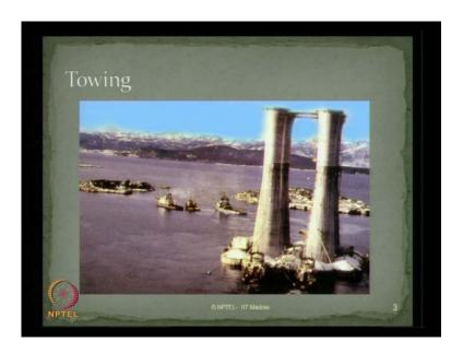
Let us quickly see some of the photographs which have been actually saying these construction and installation operations in different stages. The photograph what is see here essentially is showing, the towing of the platform with that of the boats.
