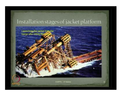
Followed by which the jacket structure is launched, so the photograph shows the launching of the jacket from the barge of the tilting the barge. So, this is the jacket template structure which is being tilted from the barge.
