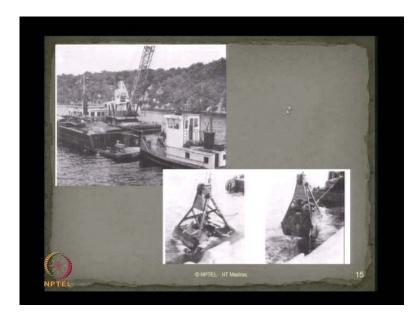
These are all photographs showing different levels of operation of a bucket dredger. As you see, the dredger is picking up the material and it is being discharged in specific form as desired.
