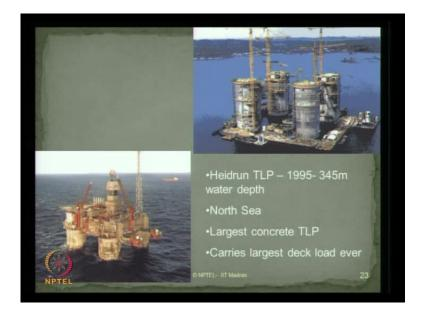
Now, let us see what is advantage of concrete being used as a material in offshore platforms? Interestingly, ladies and gentleman, Heidrun TLP, constructed in 1995 at 345 meter water depth is one of the largest concrete TLP ever constructed in the world, is located in the North sea, it carries the largest deck load ever a TLP can carry.
