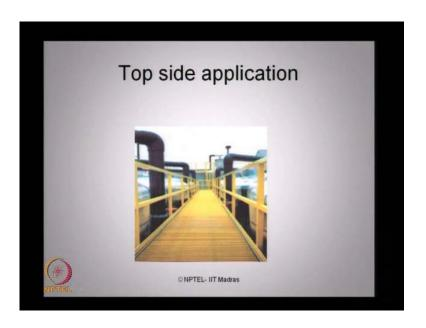
Here is a photograph which shows you the use of hand railing, grating in the pipeline where, we have used composite material as an alternative to steel.
