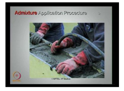
The admixture can be used directly in the shattering itself if the concrete is being poured or laid for offshore structural members.
