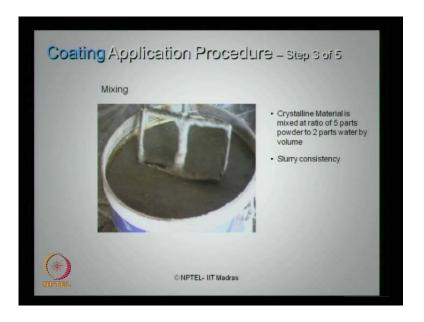
The third step in application of coating is what we called mixing. Crystalline material is mixed at ratio of 5 parts of powder to 2 parts of water by volume. Then you have to also check with the consistency of the slurry, which is formed by this mixture.
