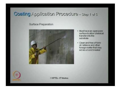
The first step is you must have an open pore surface. So, you should do a surface preparation you must have an open pore surface to allow chemical transfer into the substructure. Clean and free of form of oil, laitance and other foreign matter is essential, so that you have to do what we call a through surface preparation which will allow or admit the chemical to transfer into the surface.
