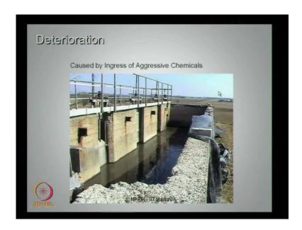
Now, what are those reasons that we can quickly focuson deterioration of concrete as a structural material. It is essentially caused by ingress of aggressive chemicals present in the environment. We have shown a photograph here, which is having a chemical reactive pond which is having lot of counter effect on the surface of a member which are essentially caused made of concrete.
