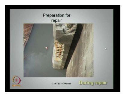
If you look at the preparation action for repair the concrete has to be completely chipped of in stages and the steel has got to be completely exposed. (Refer Slide Time: 25:08)
