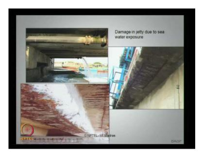
If you look at the damage picture of the jetty due to sea water exposure, again you can see here the bottom surface of the slab is also getting exposed, whereas the reinforcement is getting exposed to a severe attack of chemical environment in marine sea state.
