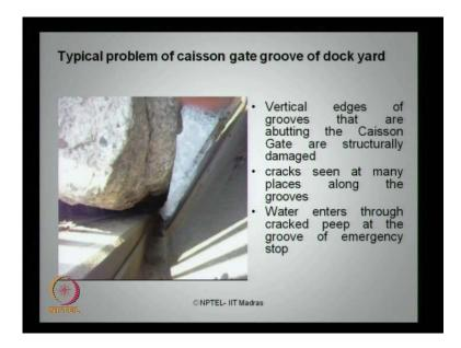
There is a damage caused therefore, waters enters through these the gates does not remain water tight. So, what would be the method to attempt a repair for this kind of treatment.
