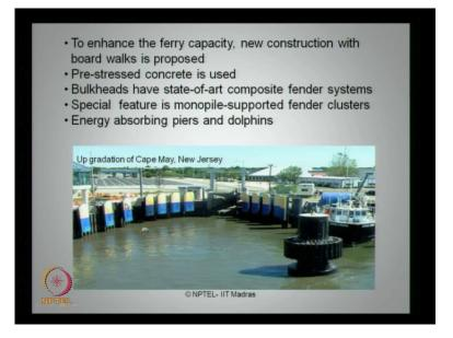
The other example what you see here, is up gradation of the Cap may in New Jersey to enhance the ferry capacity. New construction with board walks is proposed by the designer, pre stress concrete is used as a new material for enhancing the ferry capacity of this jetty. Bulk heads have state of art composite fender systems, which have been installed all along the surface special feature is a monopole supported fender clusters it, which acting as an energy absorbing piers and dolphins.
