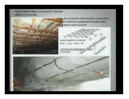
If you look at one of the examples again, where the major deterioration is caused by chloride attack on concrete. As you see here the cathodic protection which is being prepared shows a current flow from an
