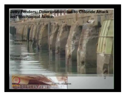
Also the jetty fenders get deteriorated due to chloride attack and mechanical action. You can see here the deteriorated jetty fenders, where the steel is getting exposed thoroughly and some repairs being attempted using a specific specification of the chemical and the concrete, which will be discussed in the next part.
