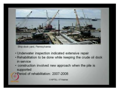
The photograph what you see here is actually a ship dock yard in Pennsylvania. The underwater inspection conducted on this dock yard indicated extensive repair rehabilitation has got to be done while keeping the crude oil dock in service, which is a very important criteria imposed on the maintenance engineer at this juncture. The construction involved actually a new approach when the pile is supported, while the loading is taking place the rehabilitation was done for this job during 2007-2008.
