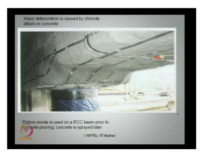
The ribbon anode is also used in RCC been prior to concrete as you see in this photograph. These are all ribbon anodes which have been used. Therefore, they are allowed to corrode whereas, the rebar inside embedded inside does not corrode because it becomes cathodic.
