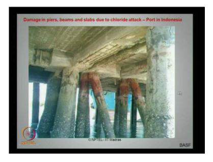
Ladies and gentlemen, it is a very interesting picture showing the damage in piers beams and socket of the slab, which are primarily due to the chlorine attack which is a port in Indonesia. You can see the socket of the beams, which are extensively corroded even the surface of the columns which are corroded and spoiling of concrete takes places, which exposes the reinforcement not only on the side faces of the beam as well as the main reinforcement in the bottom face of the beam as well.
