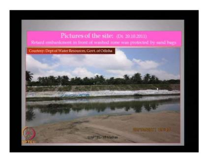
As the result of which retarded embankment constructed was completely washed the way by even though the protected by sand bags.
