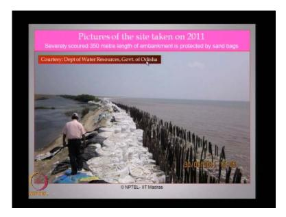
A further picture taken on 2011, which is about four years from the original problem, being noticed. You will see that the coast line has become completely merged with the land and the embankment has becomes completely ineffective about 350 to 400 meter long embankment is completely protected only by the local mechanism because of sand
