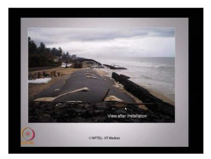
This is the one of the views after installation., these are the HDPE ropes with the gabion boxes placed in position.
