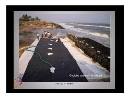
If we look at the photograph here, this is how a geo tube will be looking like before the sand is being filled in. The geo tube is being laid in the ground, and geo tube is now filled with sand you can see initially it is flat, now it is got bulge out.
