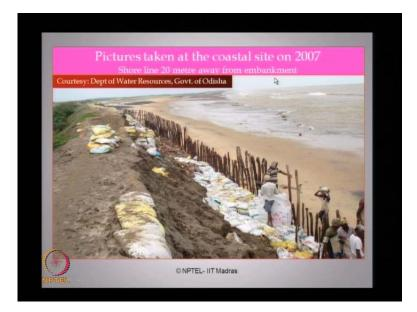
If we look at the following photograph which has been taken subsequently at different time period, for example, if you look at 2007, the photograph has been taken in the same site. The shoreline was about 20 meters away from the embankment. You can see here that is the embankment and coastal line of the shoreline is very close which is progressing towards the land where you can see here, these are all cultivable agricultural lands.
