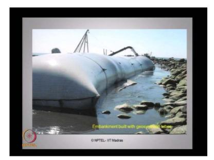
We can see here, this is geosynthetic tubes, which is filled with slurry and sand which is acting as at temporary breakwater along the groynes. The embankment which is built with the geosynthetic tubes is what you see in the photograph.
