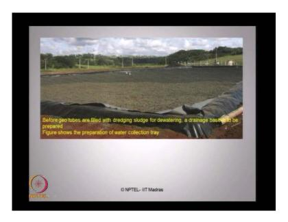
You can see here from this photograph before geo tubes are filled with dredging sludge for dewatering a drainage base as you see here need to be prepared. The figure clearly shows the preparation of a water collection tray which is got different drainage arrangement from where the drained water is taken away from the site and such arrangements are provided as long as periphery and its corner of the drainage bases.
