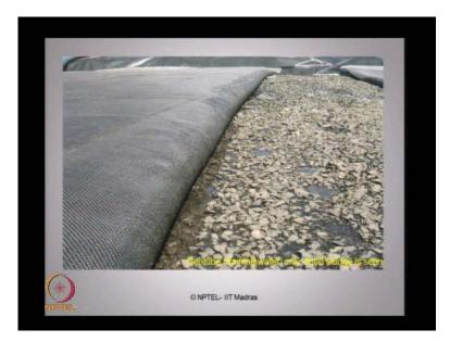
This is the very interesting photograph taken on site where the geotube drainage water is clearly seen, we can see here only the drain sludge is noted and the water has been completely percolated and drained of from the content.
