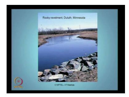
You can see here, the picture of a rocky revetment constructed at Duluth in Minnesota. You can see here basically it is less investment, is actually only a rubble lining or what we call a rocky revetment. So, the investment in terms of construction cost is not high. However, the effective functionality is also not very large compared to that of sea walls and dikes.
