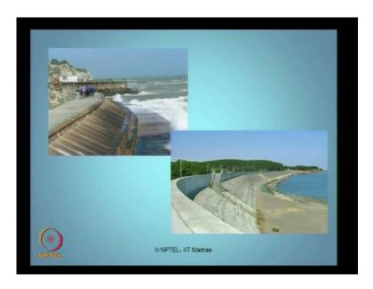
This is again a same picture, which we saw in the previous slide, is an example of a curved sea wall constructed. You can see another example here, where beautifully a curved sea wall is constructed, and the aesthetics of construction looks neat, whereas the beach is protected, but it nevertheless destroys a natural interface between the coastal site with that of the beach.
