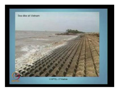
Let us quickly look at the objective of the sea dike. Sea dike is essentially constructed to prevent or control flooding by sea, on the low lying land areas. The principle function of
