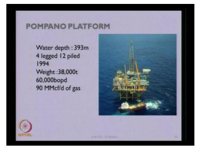
Let us talk about another kind of platform strategical information constructed in Pompano. This is the photograph of the Pompano platform constructed at a depth of 393 meters. It is a four legged platform with 12 piled free on each group constructed in the year 1994, weighs about 38000 tons. The production capacity of this platform is closed to around 60000 BOPD, which has got about 90 MMcf/d of oil, in case of the production rate.
