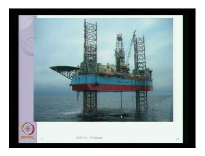
This is a closure view of one of the jack up rig, which is very famously deployed in North Sea, which is Marx Jain. This will give you a very clear picture about, how these legs are protruding the deck and how they are projecting into the sea floor as you see here.
