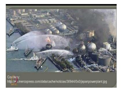
So this was the pumping sea water to the plant to control the heat.
